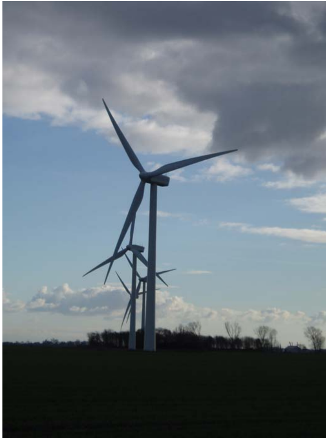
Coldham Wind Farm
