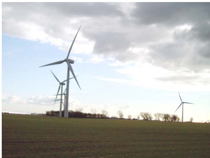
Coldham Wind Farm
