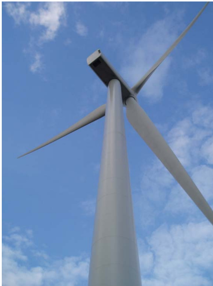
Coldham Wind Farm
