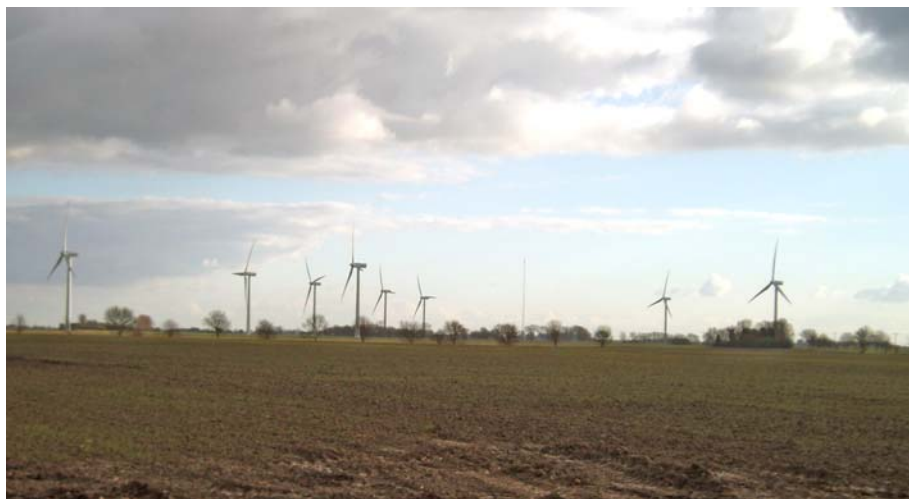
Coldham Wind Farm
