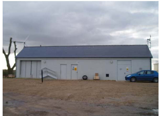
Coldham Wind Farm Substation
